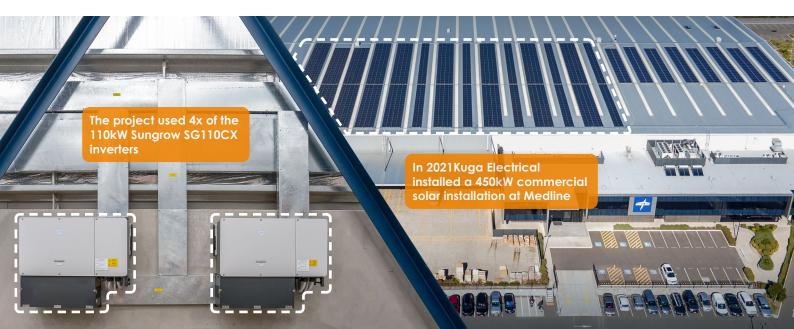
Why not use all 9 trackers on the SG110CX Inverter? It's simple. It's rare that commercial solar installations have more than 3 arrays or are impacted by shading. Usually, optimising for shade or 9 different roof orientations isn't required.
